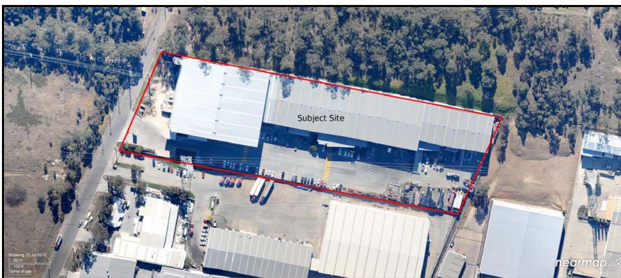
Figure 2-3: Aerial Photograph – Detailed Site View
